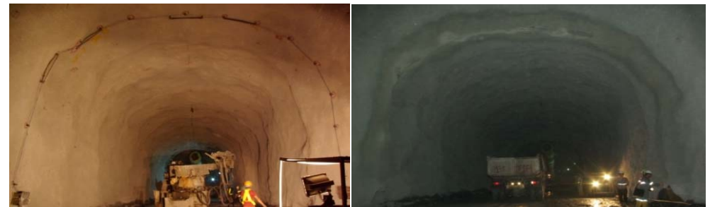
Sensor Installation : Before and after shotcreting in tunnel (AS3 Level1)
